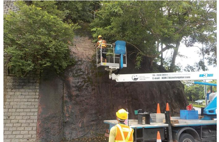
*Cleaning blocked weepholes and repairing cracked surfacing on a roadside slope*
