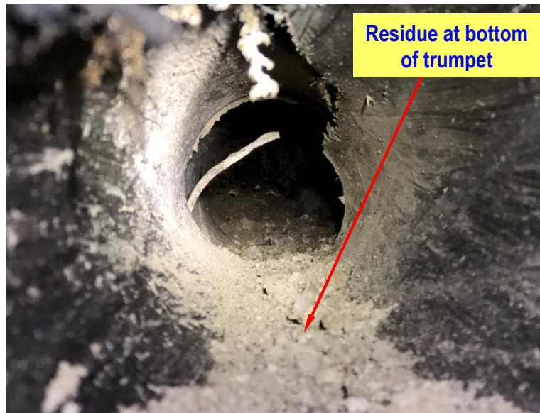
Figure 17 Residue found at the bottom of trumpet at anchor head P5
