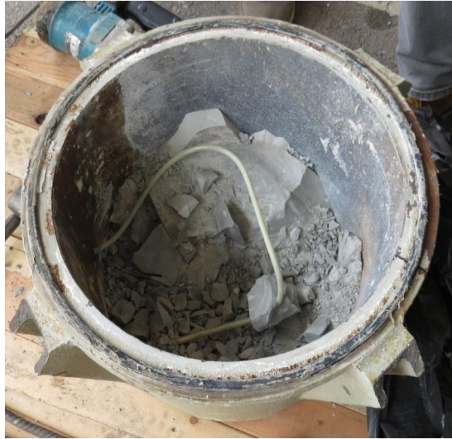
Figure 22 Condition of the air release tube at the cap of anchor head P1
