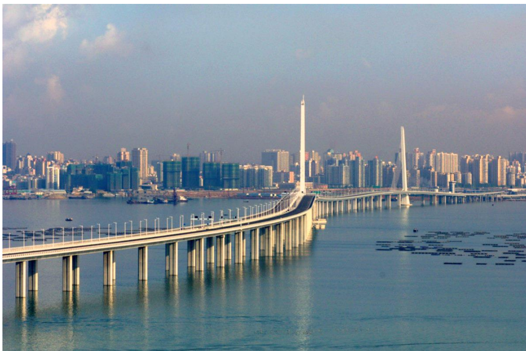
Figure 1 Overview of Shenzhen Bay Bridge
