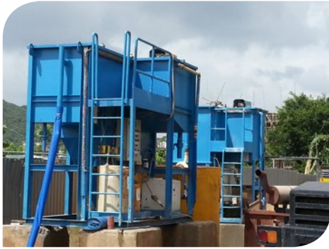
Deploy Wastewater Treatment Units on Site
