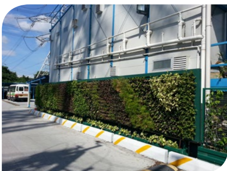
Construct Green Wall for Engineer's Site Office
