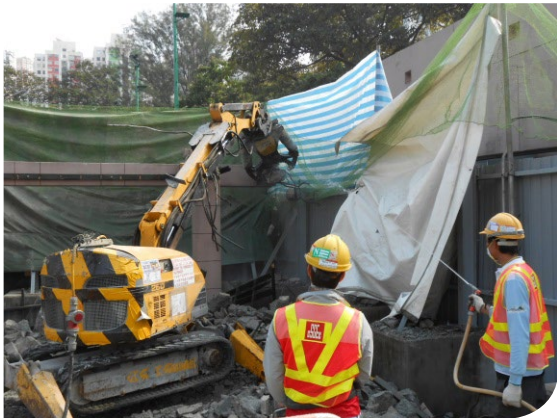
Employ Quiet Plant (Hydraulic Crushing Plant) for Pavilion Demolition Works
