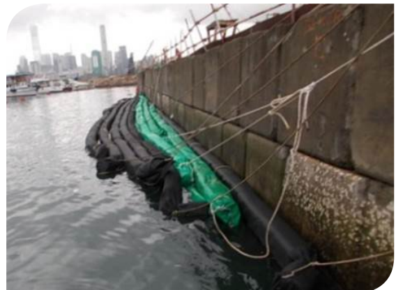
Maintain Sufficient Spare Silt Curtains and Impermeable Barriers in Stock for Contingency Use
