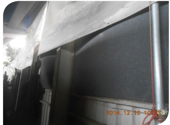
Install Noise Absorption Materials Along Site Hoarding
