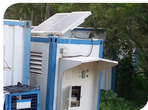
Install Solar Energy Powered Hand Key Device for Engineer's Site Office
