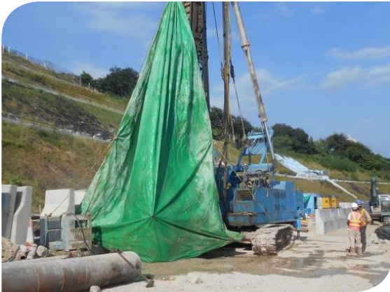
Provide Dust Screen Covers for Piling Works
