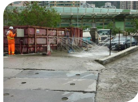
Provide Wheel Washing Facility at Site Entrances
