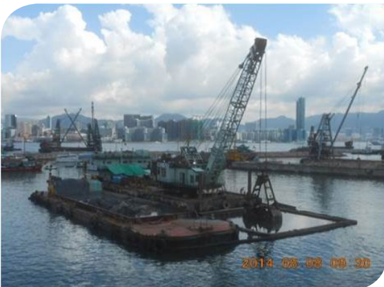
Deploy Silt Curtain for Marine Works
