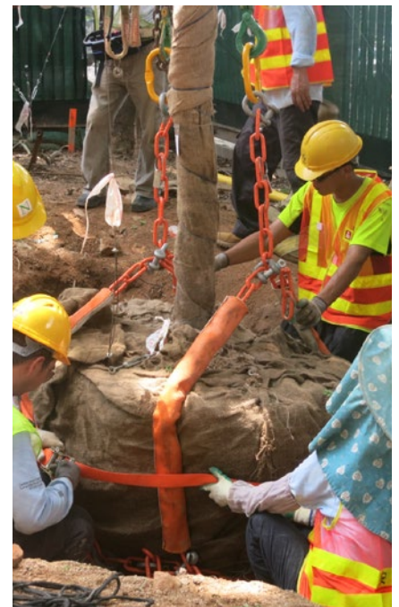
Suitable lifting gear was used to avoid any damage on tree trunks.
