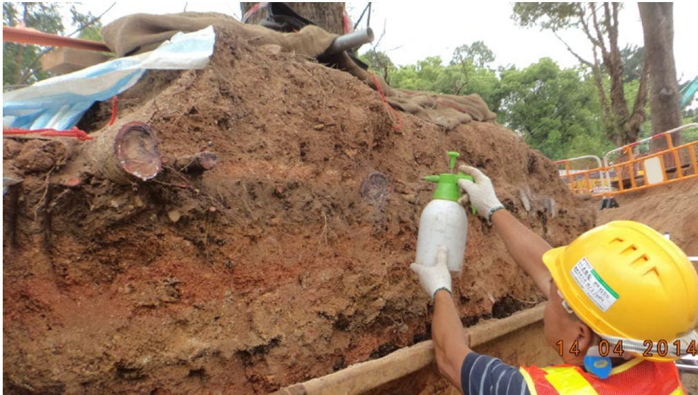
Root hormone being sprayed right after root pruning operation.
