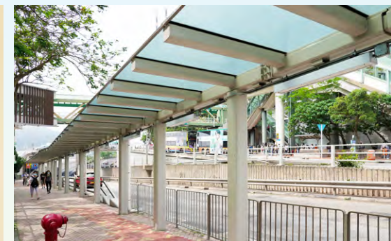
Walkway cover with laminated tempered glass panels
