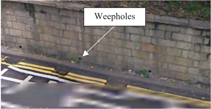
No interception channel along slope toe but holes on retaining wall
