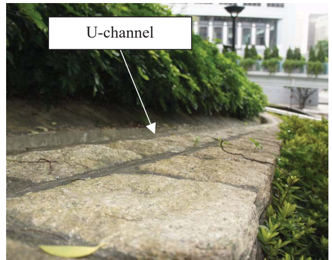
Retaining wall and interception channel
