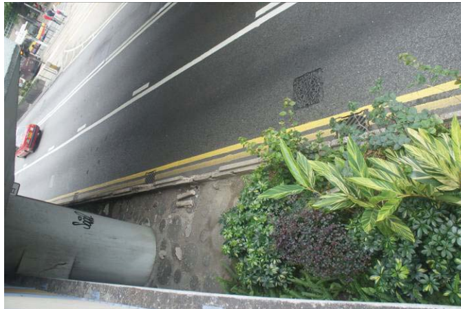
Multiple gullies near junction
