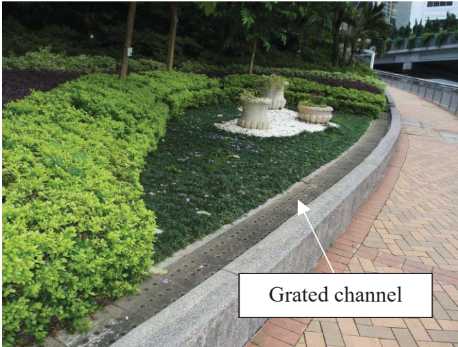
Interception channel along slope toe
