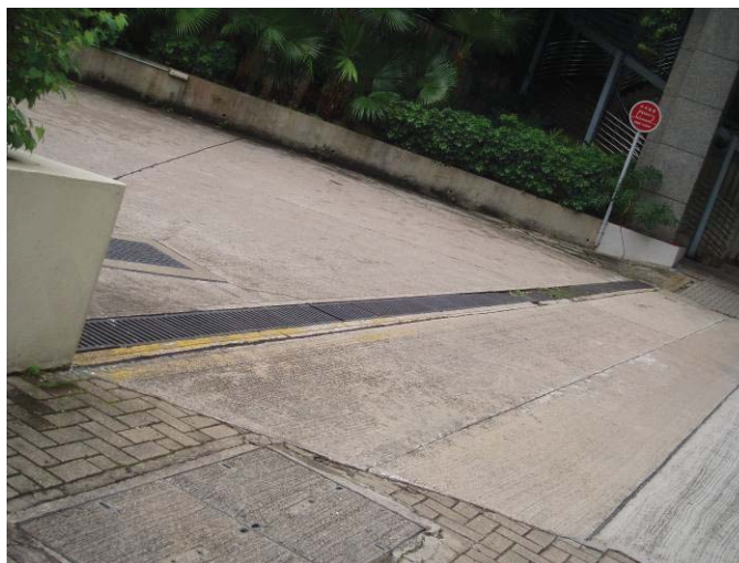
U-channel at entrance/exit of the fire station
