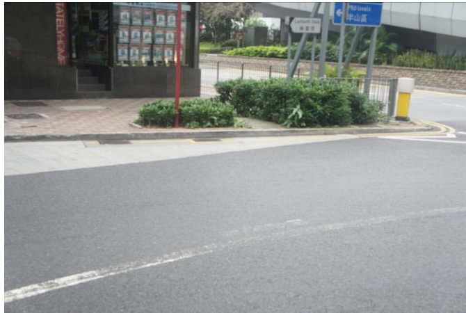
Double gullies at junction
