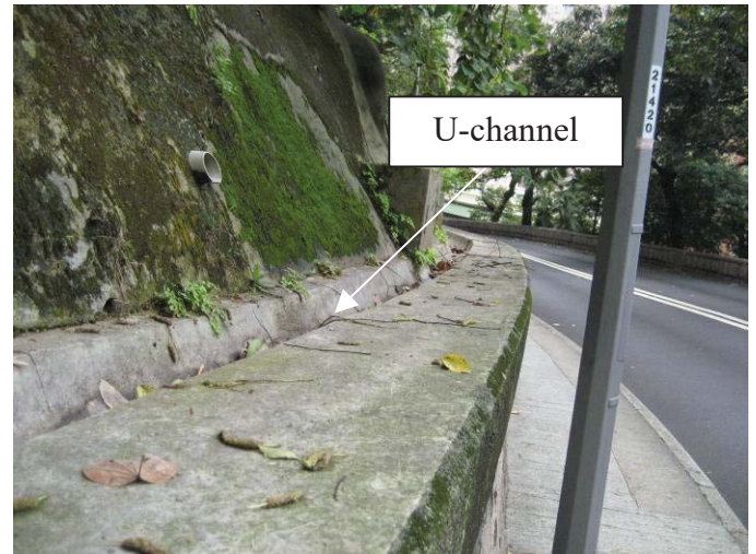
Interception channel along slope toe
