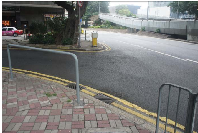
Double gullies at junction
