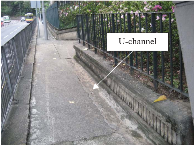
Interception channel along slope toe
