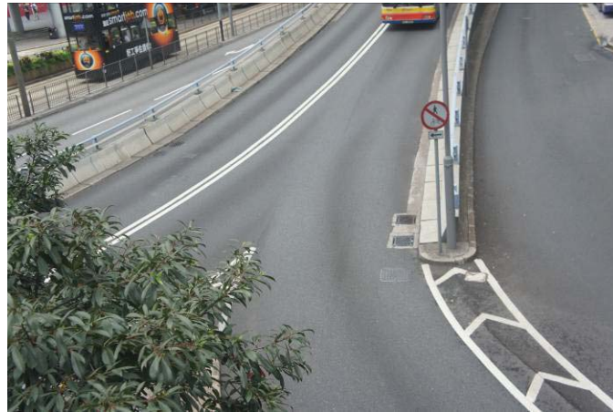
Double gullies at junction
