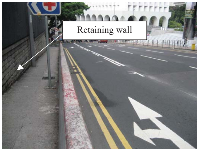
Retaining wall at slope toe
