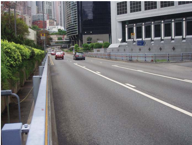
No gully on a long section of road pavement
