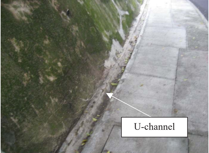
Interception channel along slope toe
