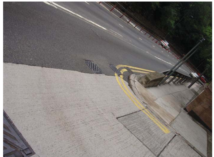
Multiple gullies near the junction
