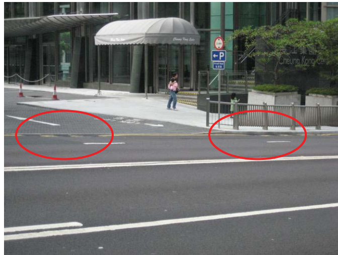
Multiple gullies at entrance/exit of the development
