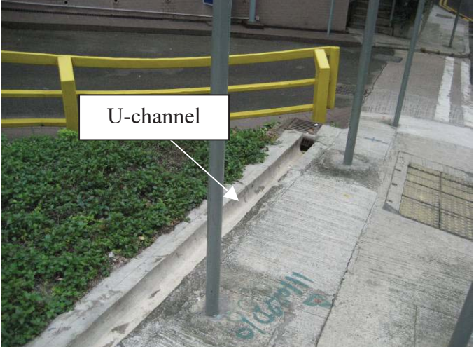
Interception channel along slope toe
