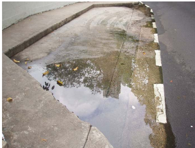
No gully or channel at lay-by
