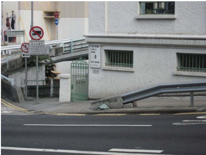
Multiple gullies at junction
