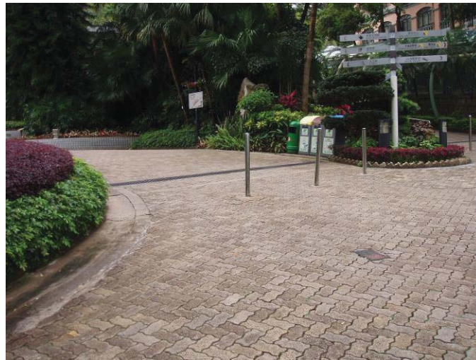
U-channel at entrance/exit of the park
