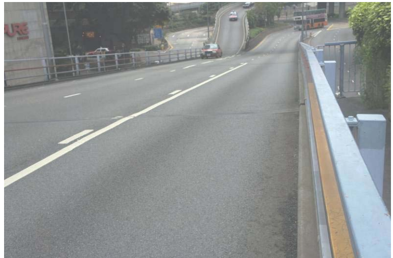
No gully on a long section of road pavement
