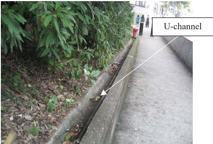
Interception channel along slope toe
