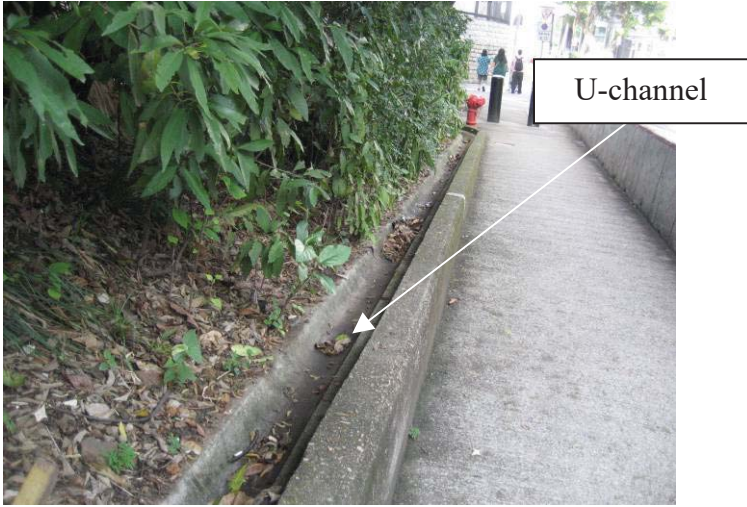
Interception channel along slope toe
