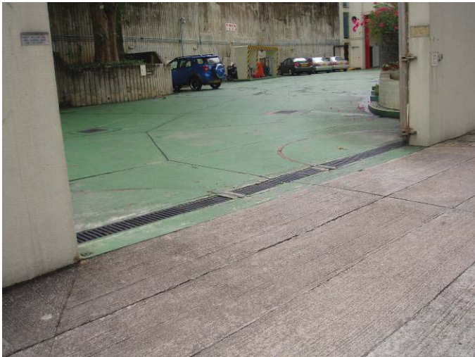
U-channel at another entrance/exit of the fire station
