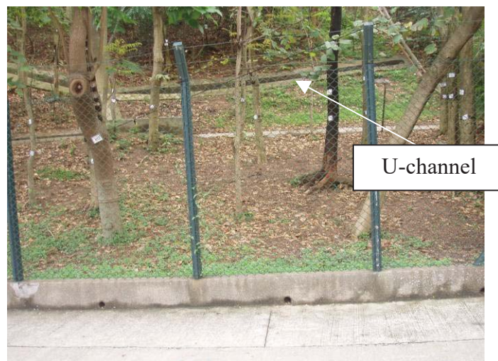
Interception channel at mid-way but not along slope toe
