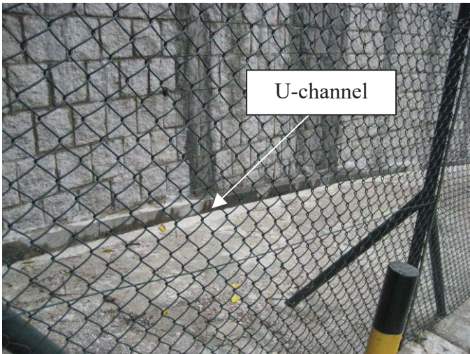
Interception channel along slope toe
