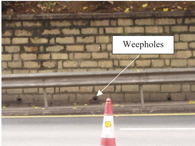
No interception channel along slope toe but holes on retaining wall
