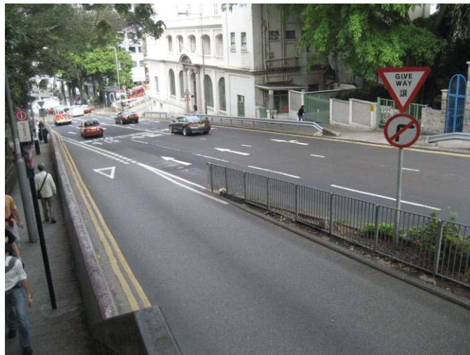
No gully near the junction
