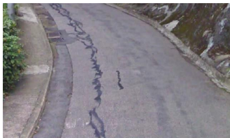
Photo 2 – Filling of interconnected cracks on a low-volume rural road
